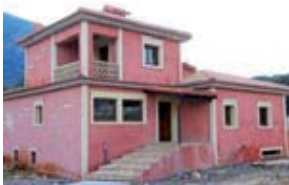
Bioclimatic house in Sami, Kefalonia (Greece). The house is one of the very few Ecological/Bioclimatic buildings on the island.
