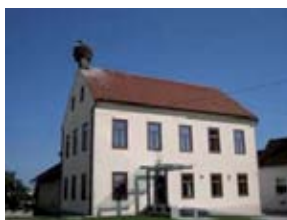
Smart house, Martjanci, Lea (Slovenie). XVIII century old building renovated with bioclimatic criteria.
