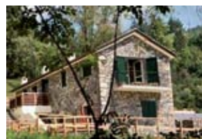
Farm holiday renovation, “Centro Anidra”, Borzonasca (Genova, Italy). Use of materials / technologies from local traditions and renewable energy.
