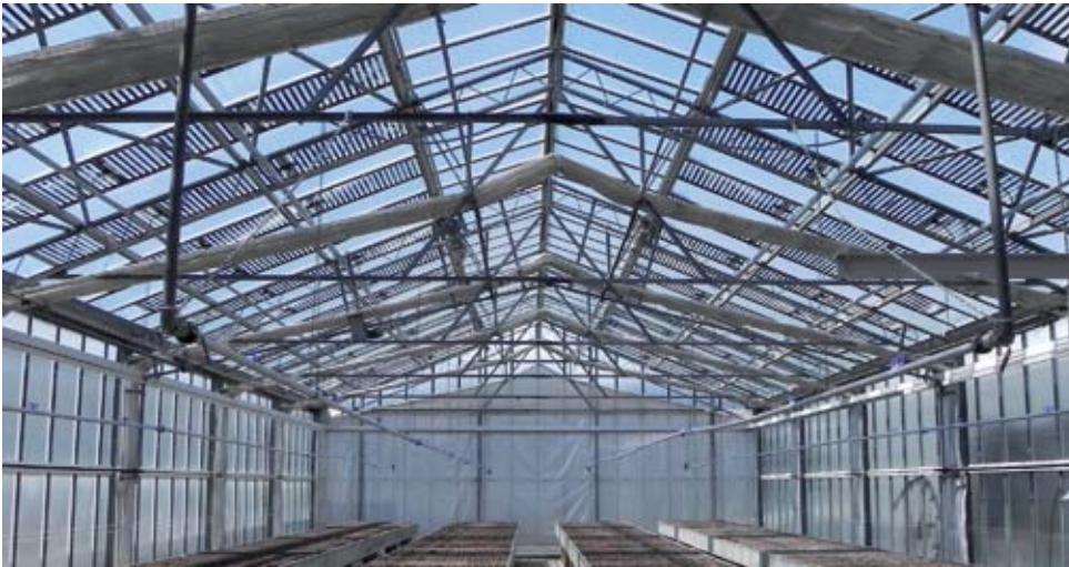
One of the case studies that were examined: Integration of innovative photovoltaic systems on the agricultural greenhouses of CerSAA in Albenga (SV).
