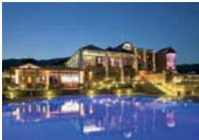
Regina dell'Acqua resort, Skala, Kefalonia (Greece). Five star hotel constructed according to the rules of sustainable building.
