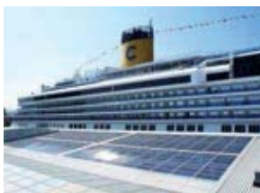
Terminal Costa Cruises, Savona (Italy). Rooftop photovoltaic in harbour area.
