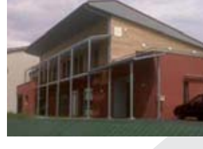
Parc eco-habitat, Saint Symphorien sur Coise, Lyon (France). Public Building Green Construction.
