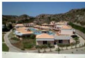
Hotel "La Marquise"(Greece). Complex hotel with smart energy management system.
