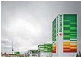
Heineken Brewery , Sevilla (Spain). Energy optimization in industrial building.
