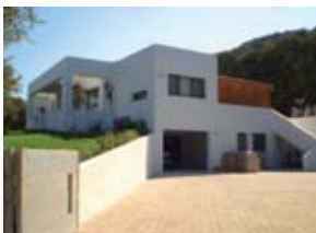
Private house in Ialissos (Greece). Sustainable building.
