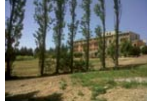
Monastery of Vaugneray, Lyon (France). Eco refurbishment of a monastery into housing.
