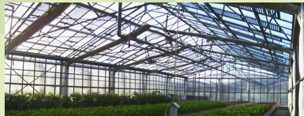
Double purpose greenhouse with panels CIS (Copper Indium Selenium)
