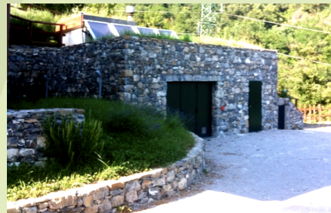
Building and equipment house built into the terraces. In the thermal power plant: wood-fired boiler and storage tank. On the green roof: solar panels (mq 8)
