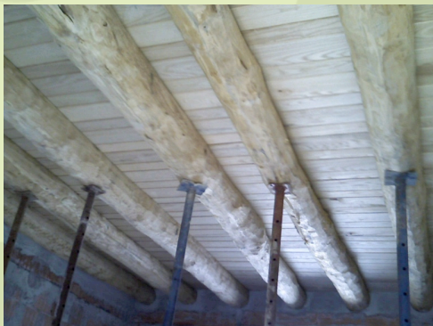
Using the wood: chesnut floors, wood fiber insulation board mineralized, willow railing
