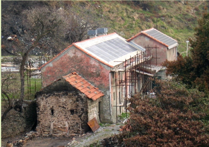
Genova Pegli: integrated photovoltaic tiles in the mantle slate - project arch. P.Rissotto
