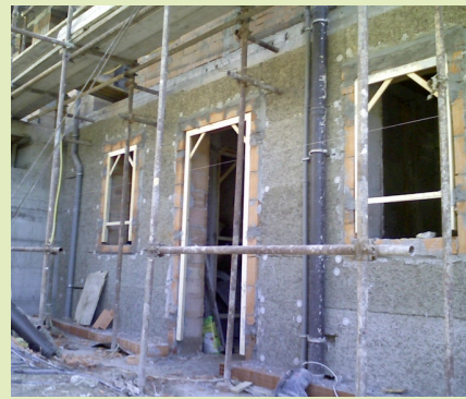
Using the wood: chesnut floors, wood fiber insulation board mineralized, willow railing
