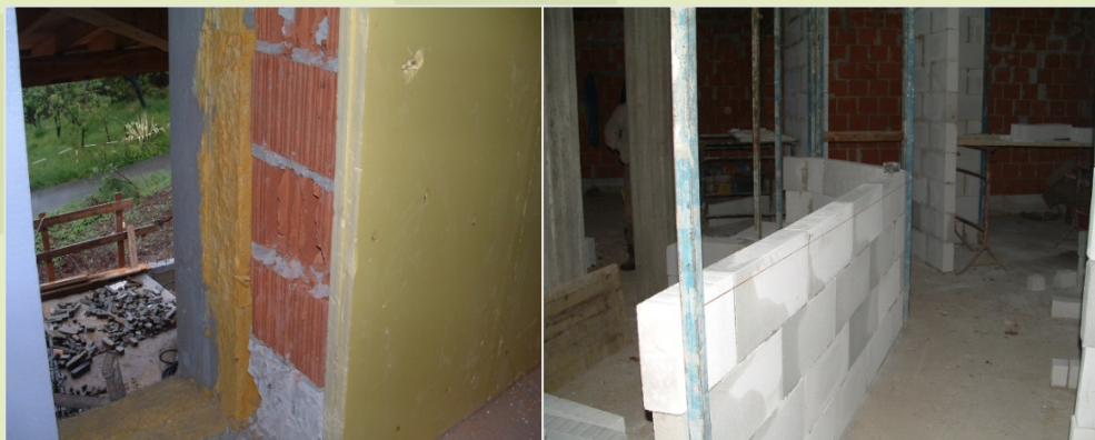
Natural stone cladding, partitions gas concrete, insulation bearing masonry, lime plasters, low-emissivity glass
