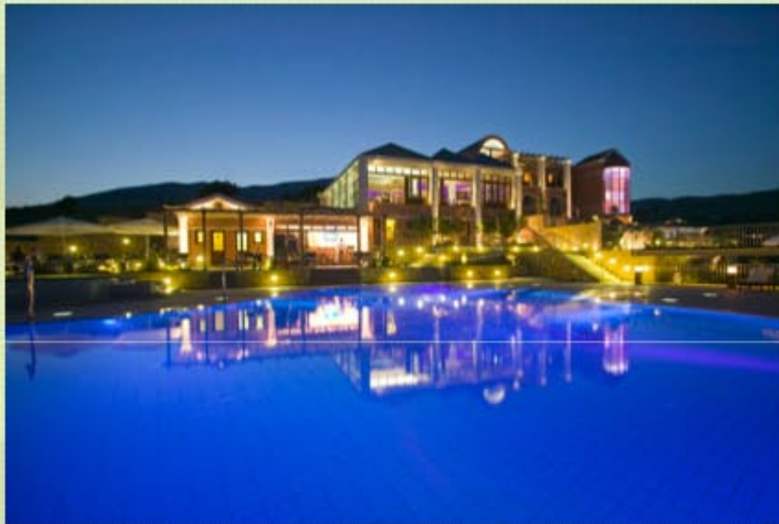
The large windows and sun shades of the hotel
