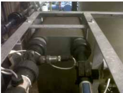
Plate heat exchanger
